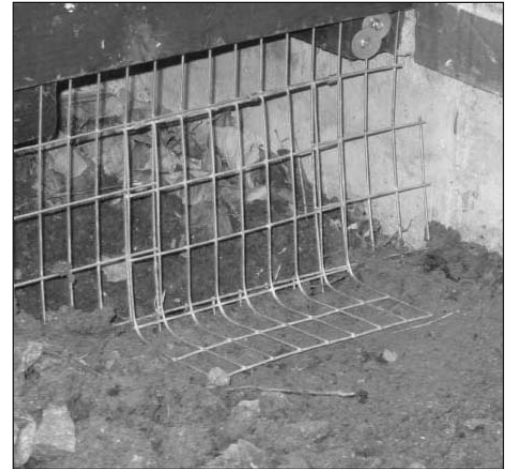
This 1-way door fits under a deck to let raccoons, skunks or cats out and can easily be made on the spot.
